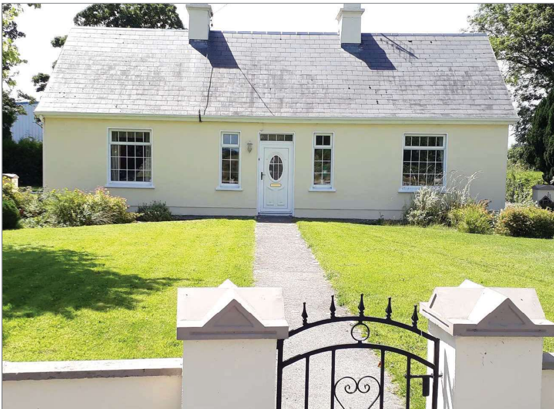
Illus. 5.1 and 5.2—Two attractive, well-maintained houses with traditional features are directly threatened by Route Option 2 (Inventory No. 15, above) and Route Option 3 (No. 18, below) and would be demolished, amounting to severe impacts of these options.
